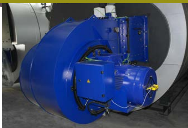
TEMINOX GL in use on a flame-tube and a double flame-tube boiler
